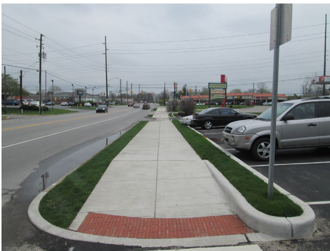
FIGURE 12: EXAMPLE OF STREET-LEVEL CROSSING WITH MARKED CROSSWALK
